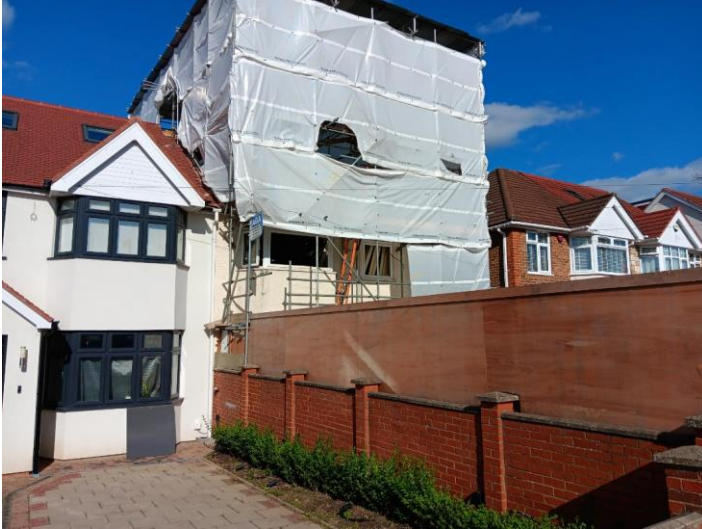
Figure 3 Front of property and adjoining semi-detached unit
